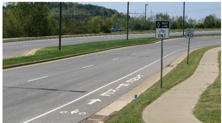
Typical bike lane with signing and markings
