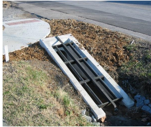
TDOT Safety Endwall
