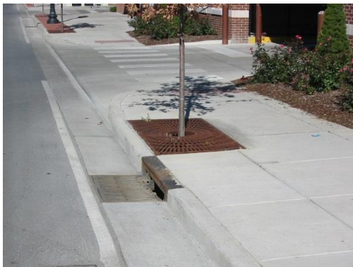
Vertical combined curb and gutter
