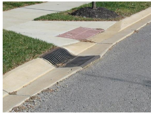
Rollover curb with grate transition
